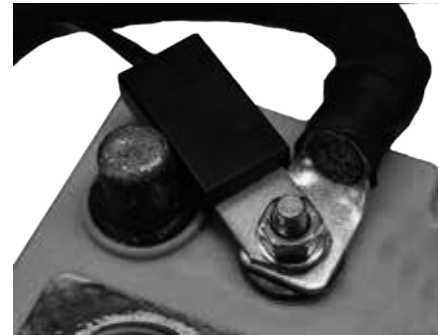
Fig 2.5(b) Temperature Sensor Installation
